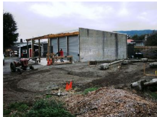
Clearing the site and laying out the poles
