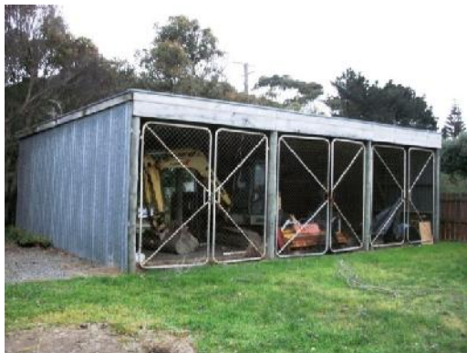
Tractor shed that was dismantled
