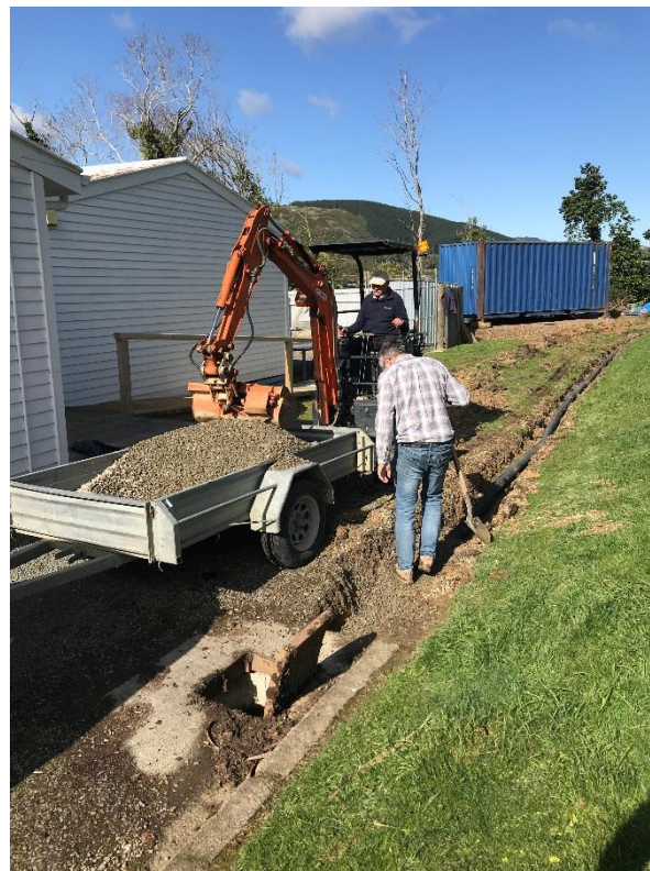
Ron Lucas and Graeme Blick did an amazing job to trench, drain and gravel the mud swamp leading around to our gardens.
