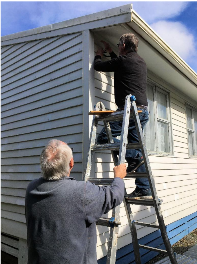
Richard and Murray instal a new security light.
