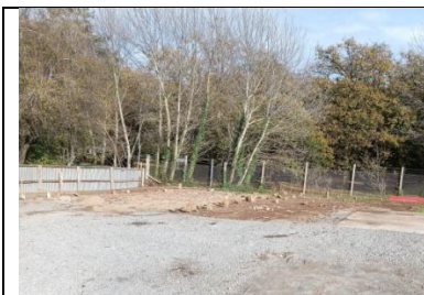
21 st April. Site cleared.
