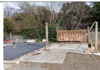
21 st April. Site of Sutton's Office- BBQ areas cleared.
