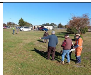
23 rd April. Laying out the pegs for the new buildings
